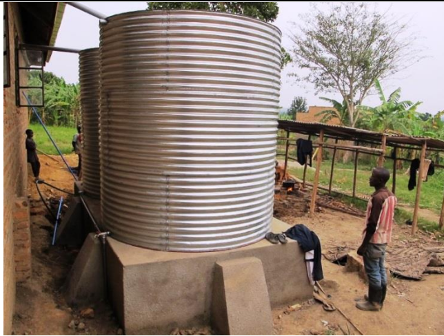
The galvanized rainwater harvesting tanks
