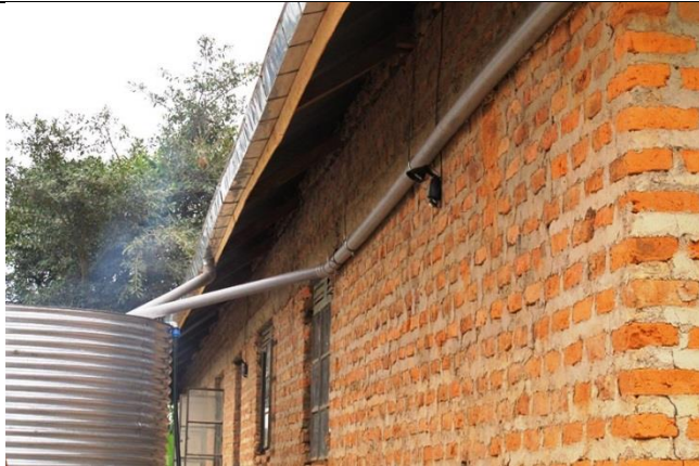
Gutter, pipes and solar light
