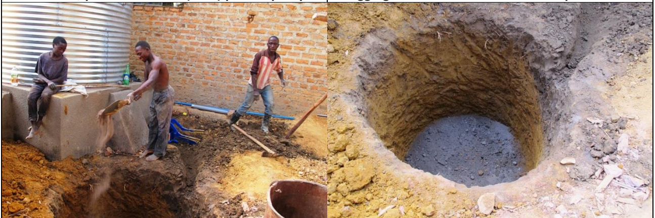
Making a "soft" bed for the plastic tank
