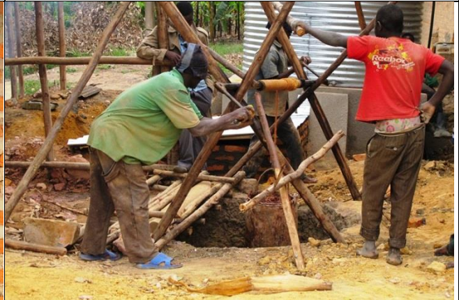
Towing up bucket with soil and stones
