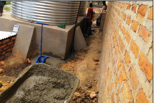
Making a slab for peddle pump and tap on tank
