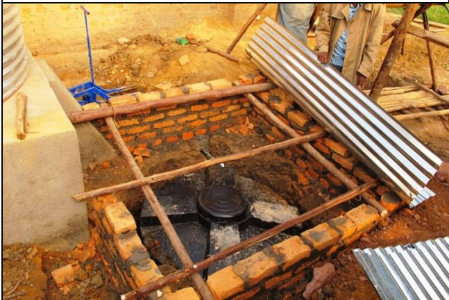
Making a cover of bricks and iron sheets
