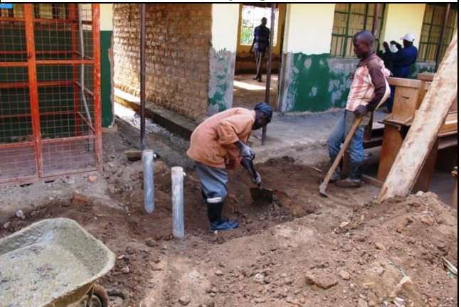
Slab in front for clean water taps
