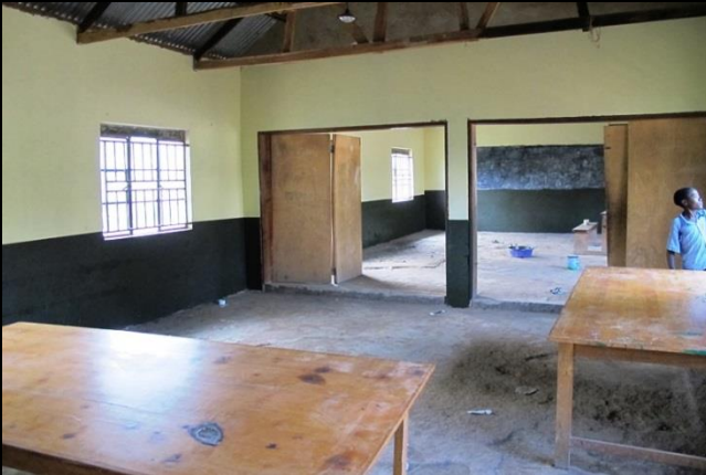
Main Hall to be ready, but still to be cleaned
