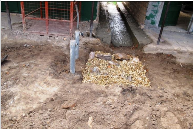
Needs proper foundation
