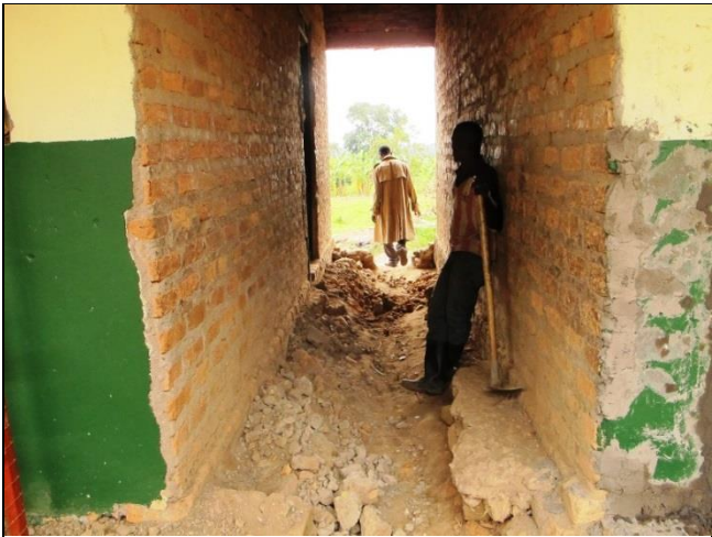
Cutting out the dangerous areas
