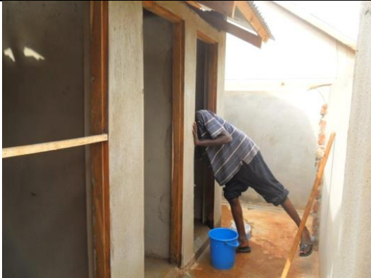
Frames of the doors being fixed in the toilets.
