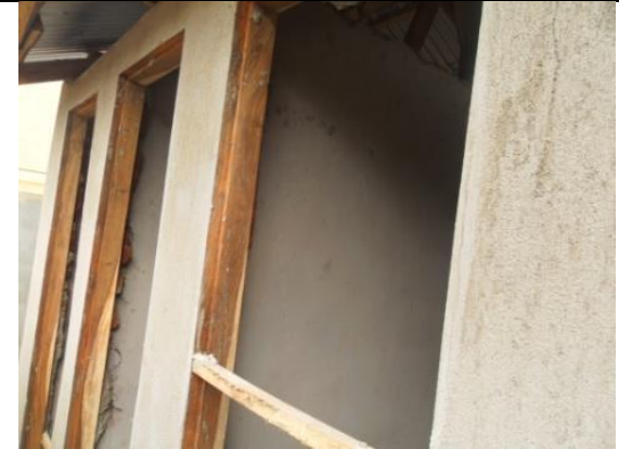
Door frames of the other side of the toilet also fixed in.
