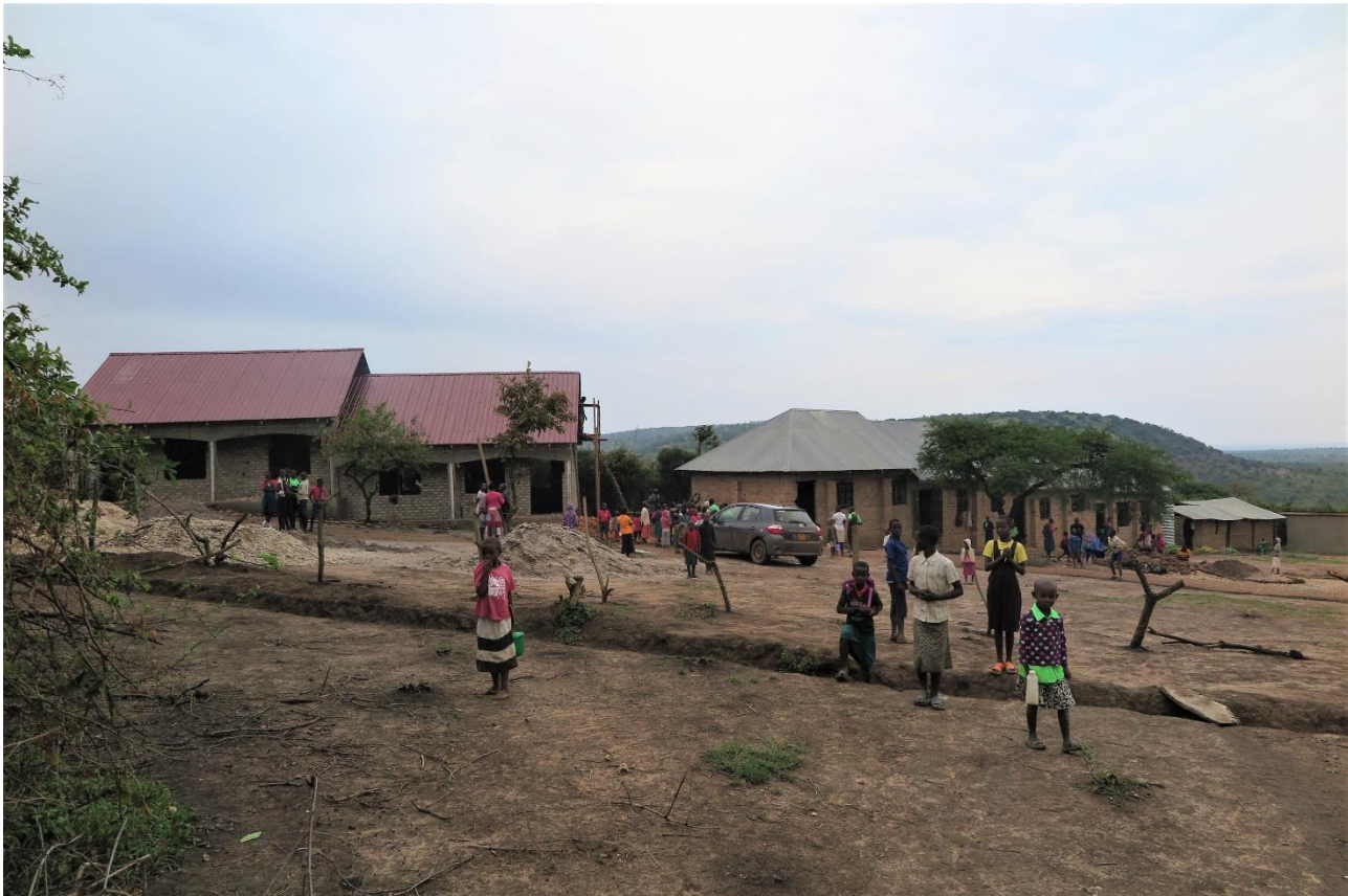
Construction of 2 Class Rooms in September 2017
