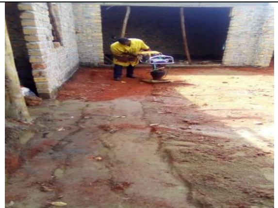
Levelling of the compound to make the parking area at the front of the restaurant
