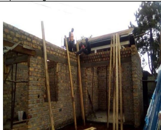
Timber for starting roofing works
