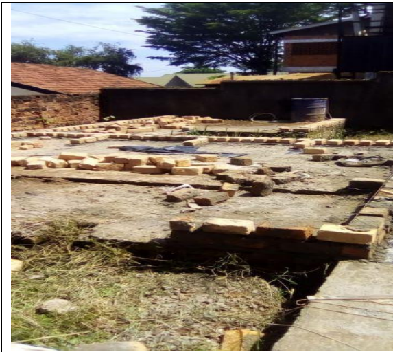
The foundation slab
