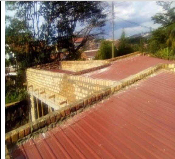
Roofed structure is complete
