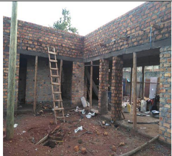
Parapet wall ready for plastering works to start
