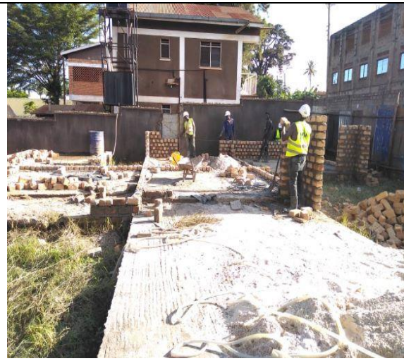
Builders start raising the walls
