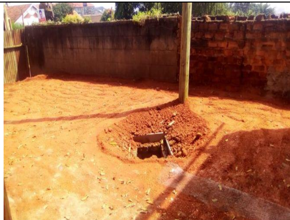
Back side of the building filled with soil, green grass will be planted here. The hole is a manhole (with drainage pipe) which will be covered.
