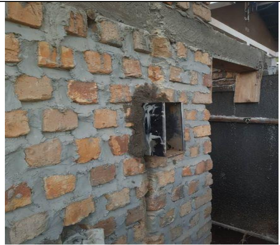
Outside electricity metre box shell
