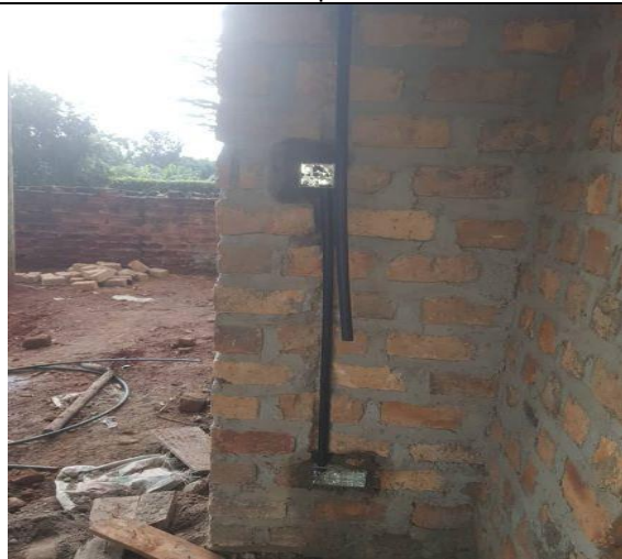
Some of interior electrical works
