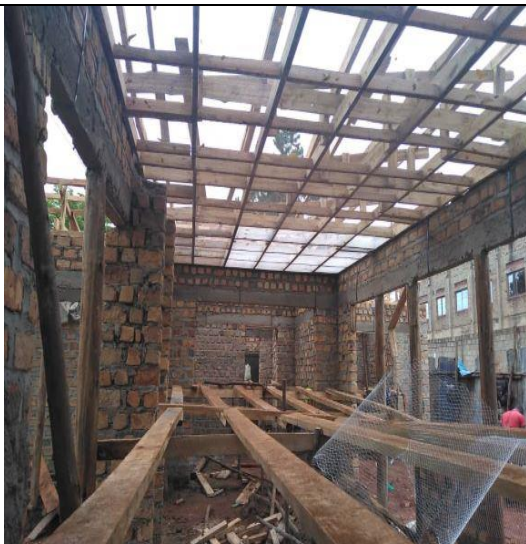
Timber and wire mesh for making roof and ceiling
