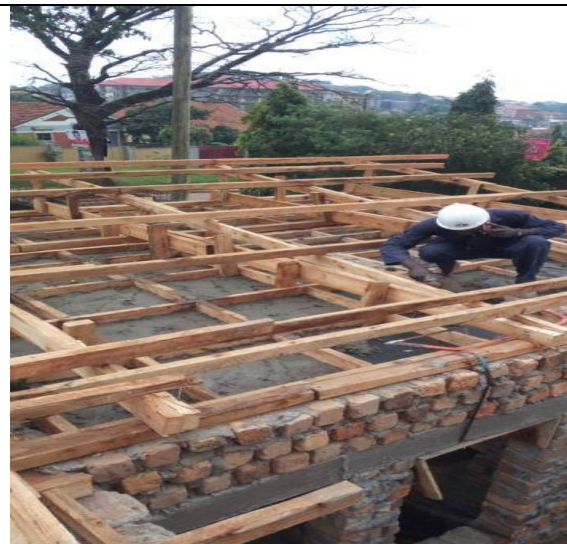
Builder roofing the building
