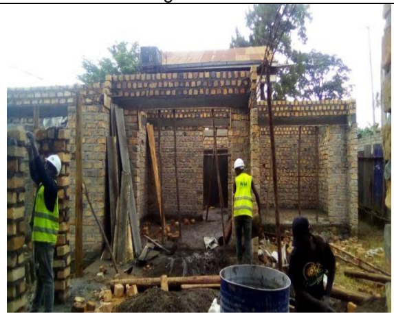
Builders build up to the beam level
