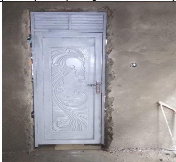
Back evacuation door is fitted
