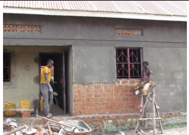
Workmen plastering and fixing windows
