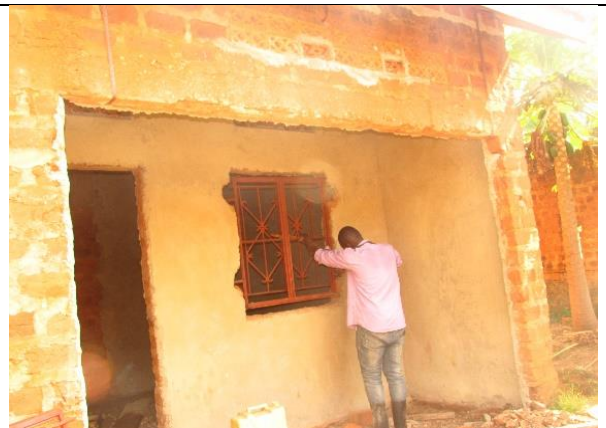
During the progress and the current state after the project
