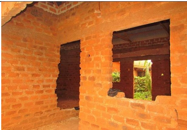
Original state of the building
