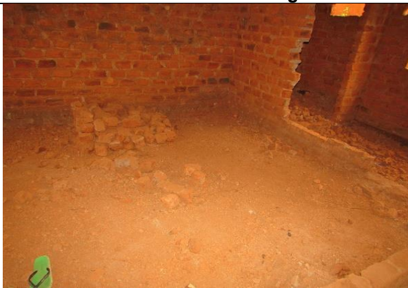
The original floor is soily and dusty
