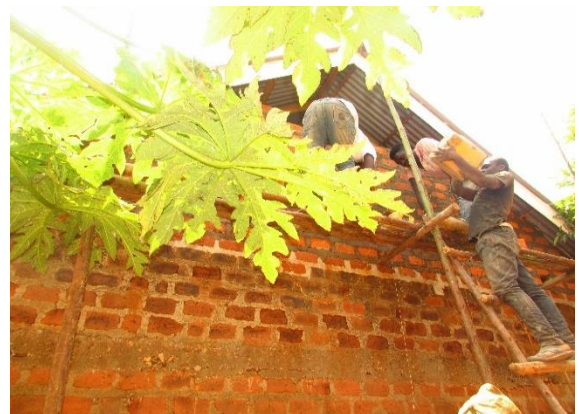
The walls have been raised
