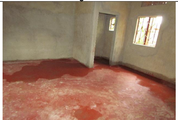
Flooring of the building is now ready
