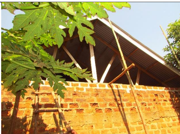
Before raising walls
