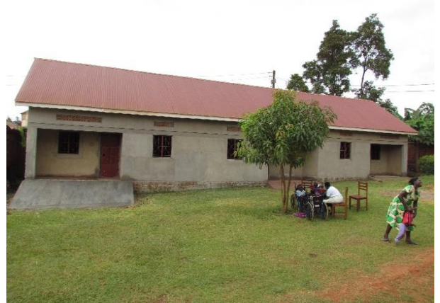
The front of the building is now plastered. Entrance has been made with a ramp to accommodate entry of wheel chairs.
