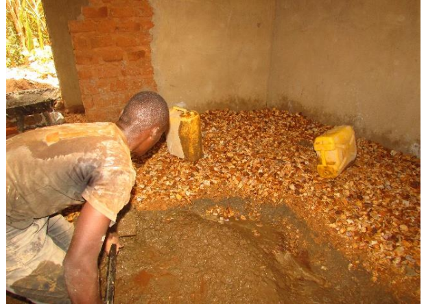
Making the floors
