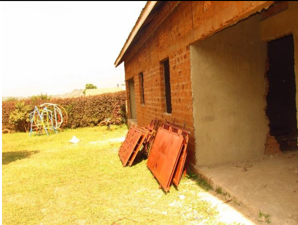
Before fixing windows
