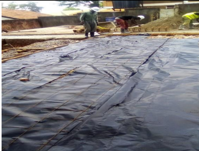
A very strong foundation for the building was laid.
