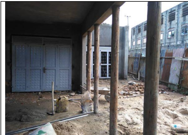
Doors and windows were fitted
