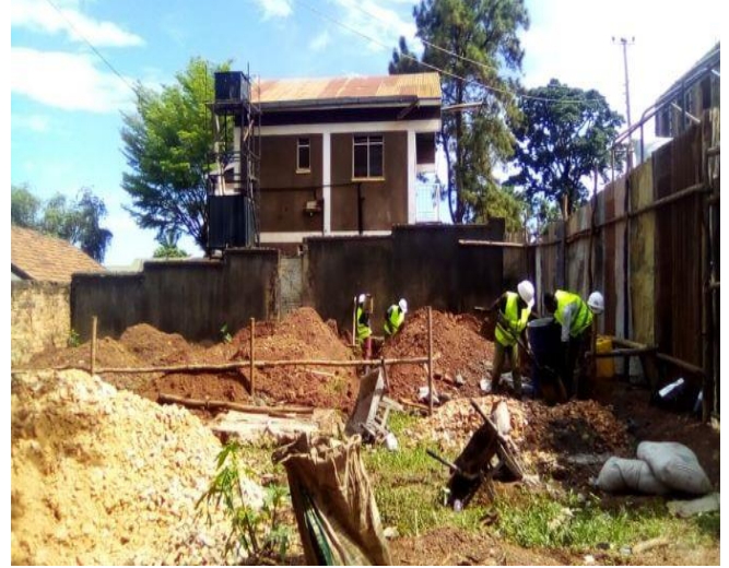
Setting out and digging to lay the foundation
