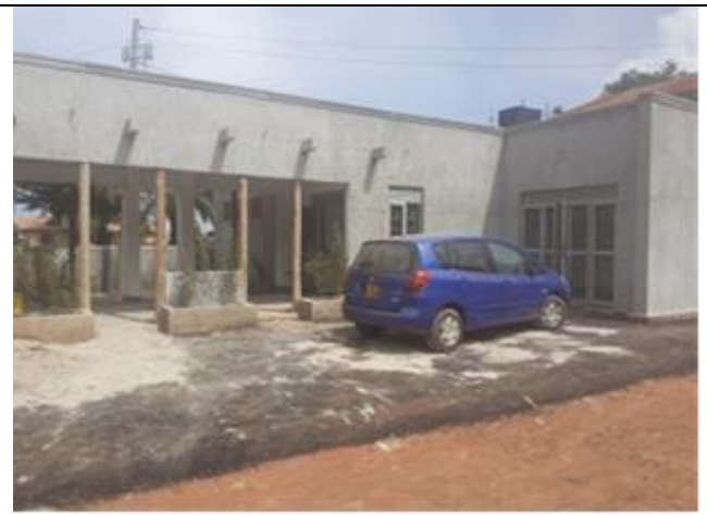
Plastering of the walls is done
