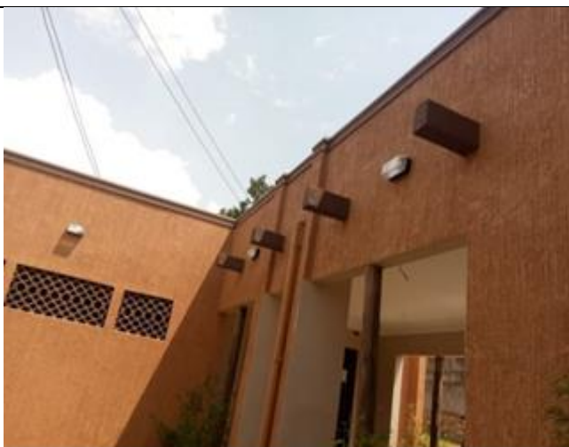
Electricity installations are done and the building is surrounded by security lights as shown above
