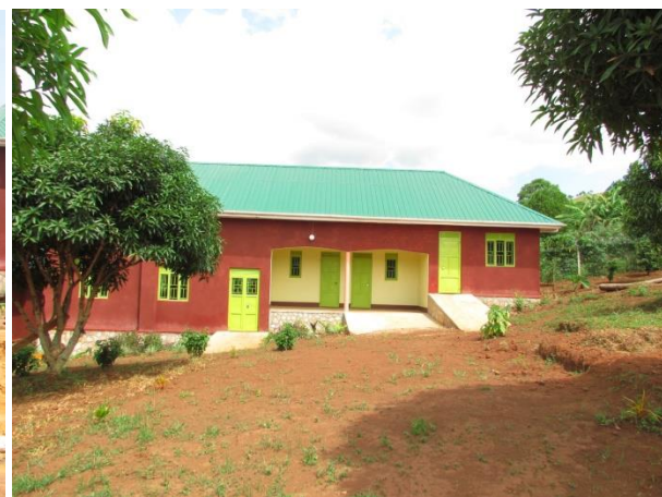
Administration Block and library
