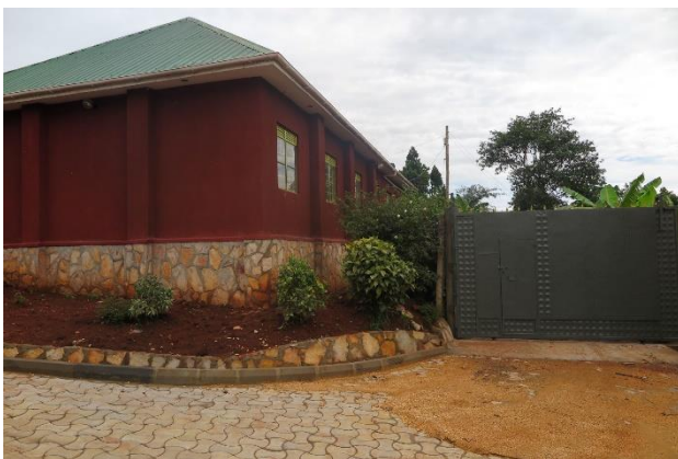
Well-secured entrance with electricity supply
