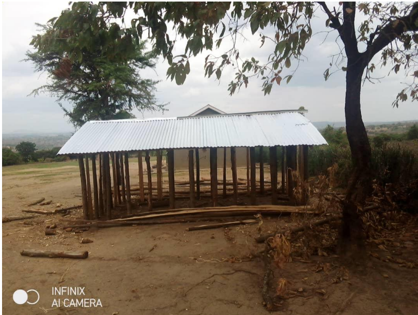
Chicken shelter construction in progress
