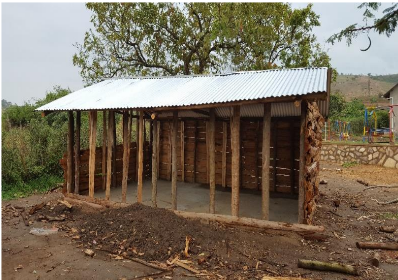
Chicken shed under construction
