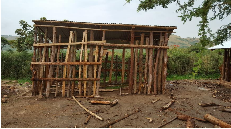
Cow shed constructed
