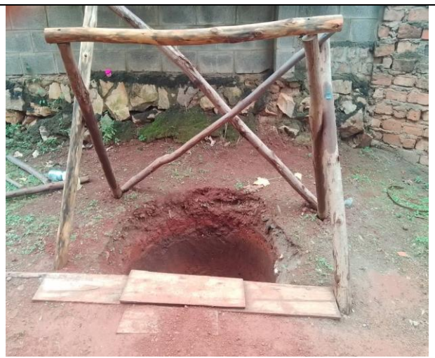
Protected drilled well before construction
