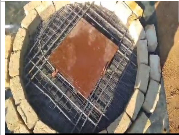
Construction of the slab to cover the well
