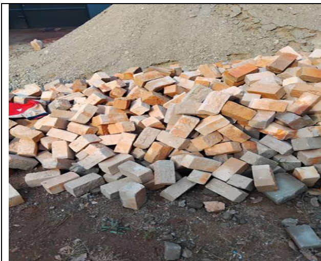
Sand and bricks for the construction of concrete walls and slab
