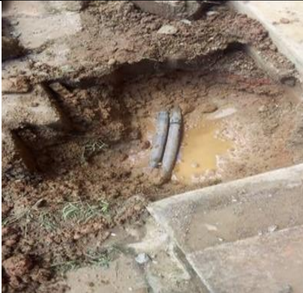
One of the connections made to the restaurant
